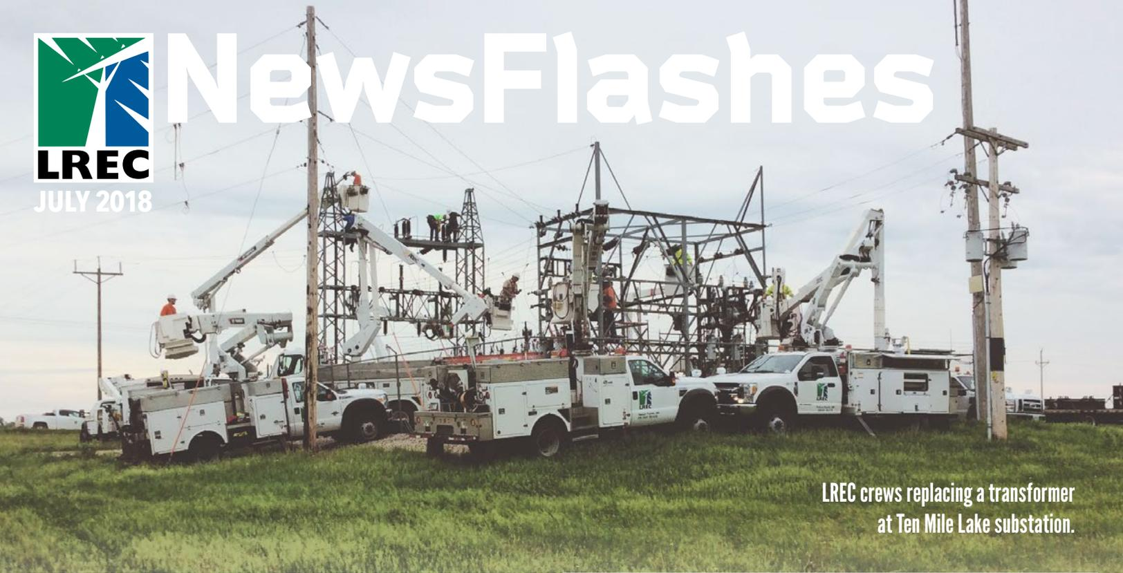
LREC crews replacing a transformer at Ten Mile Lake substation.
