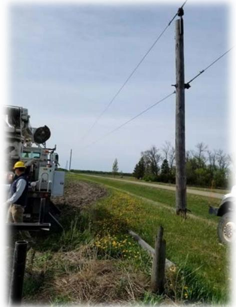
Operator of equipment hit pole, snapping it in half but lines remained in the air
