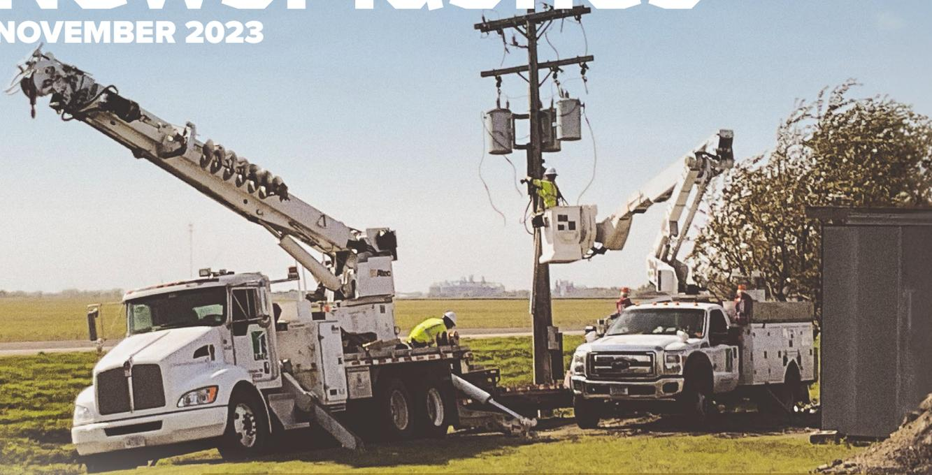
LREC crews switch out poles and eliminate overhead wires for a new substation switch to be installed by our power provider, Great River Energy. The high voltage transmission switch provides the Ten Mile Lake substation with power.
